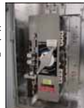
Automatic Transfer Switch
