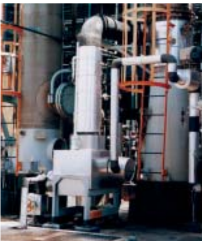
Compabloc installed as stripping column reboiler at an ethyl-acetate plant in Rhodia, Brazil
