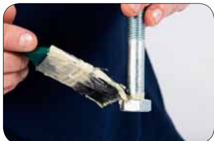
7.1 Grease the tightening bolts and nuts.
