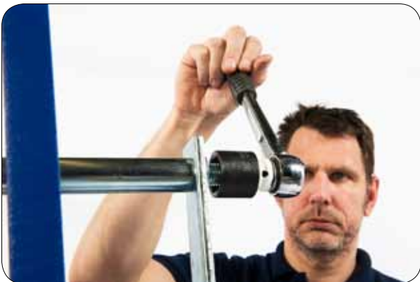
9.2 Fasten the bolts to secure the support column.
